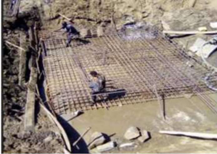
Fig 1: Construction of 3 span bridge in along kusijoni-Eribaku Road, Adjumani
