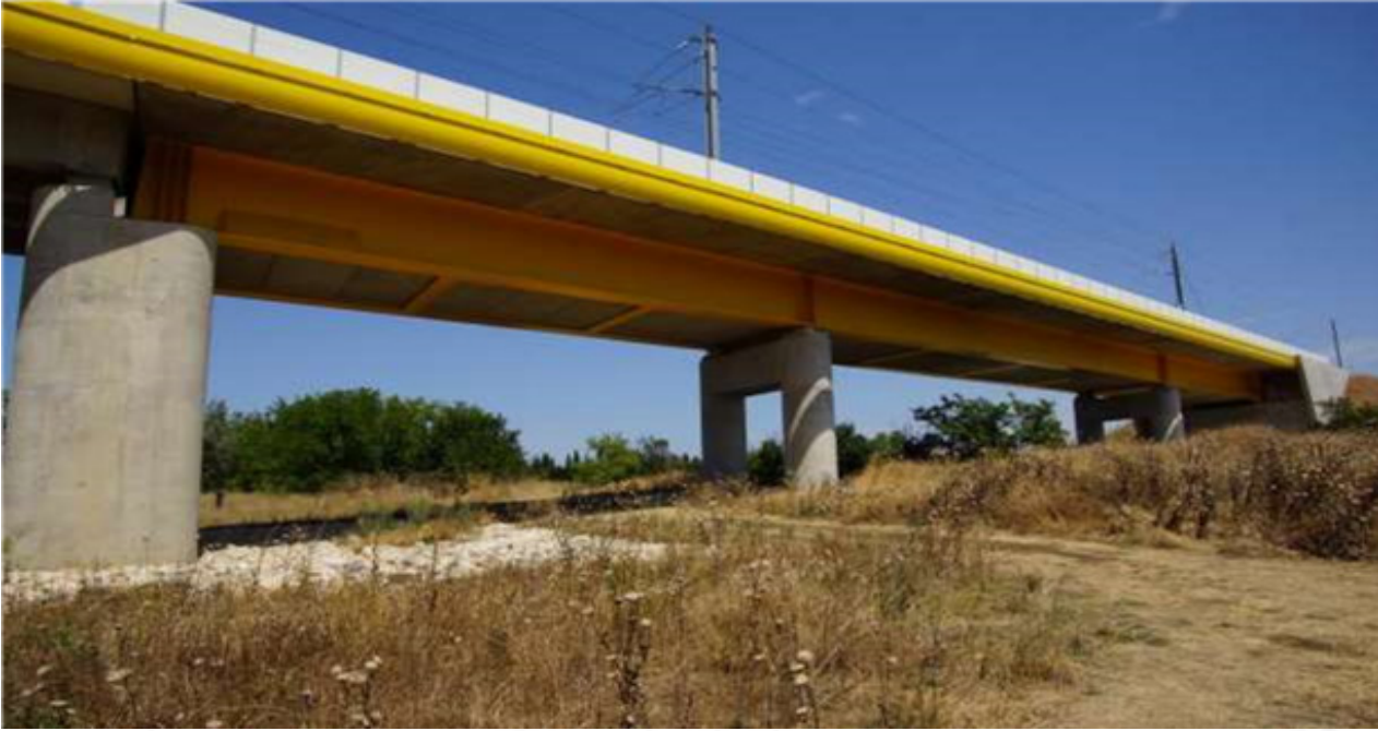
Fig 6: Completed 3 Span Bridge along Kusijoni-Eribaku Road, Adjumani
