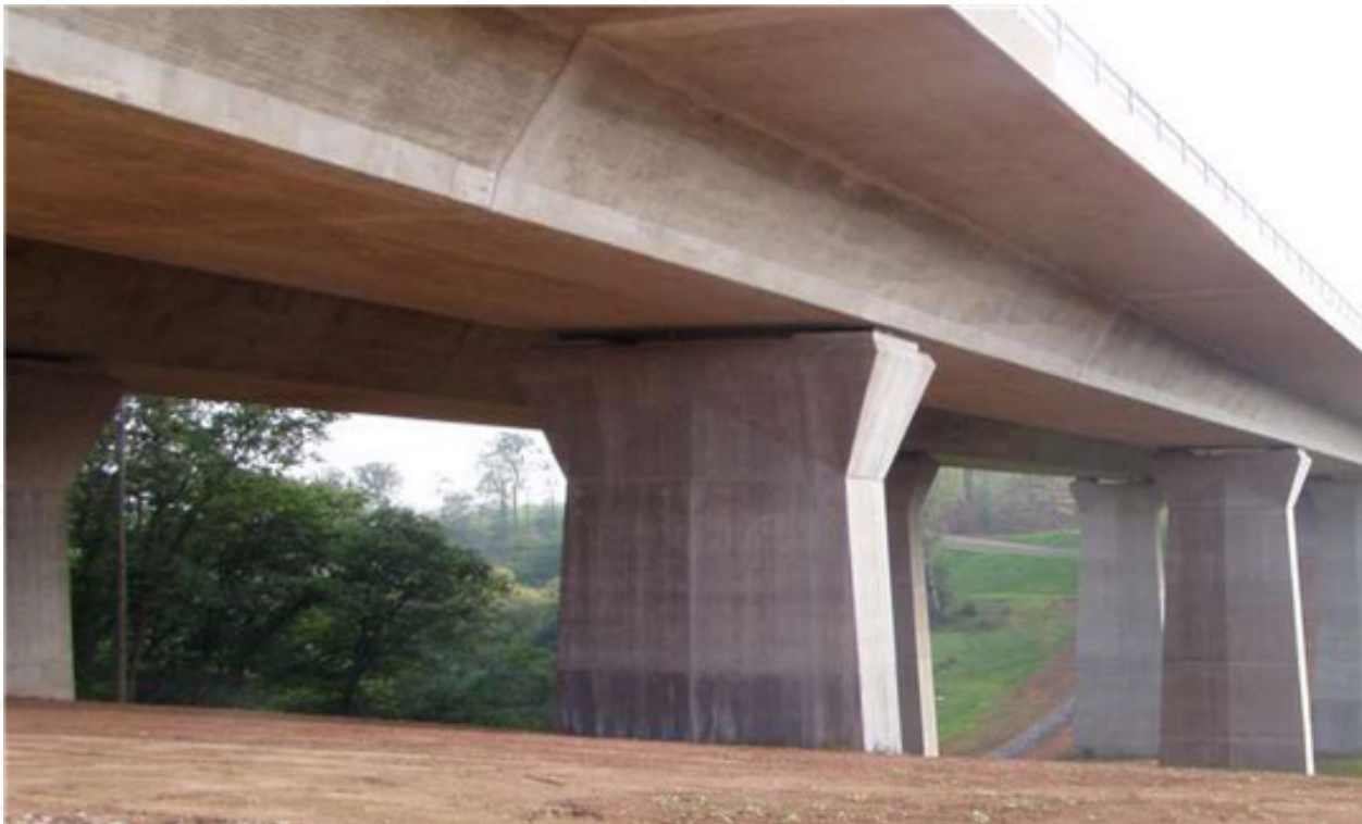
Fig 7: Completed 3 span bridge at Monroc Market – Owak-Bungatira Road Gulu district.
