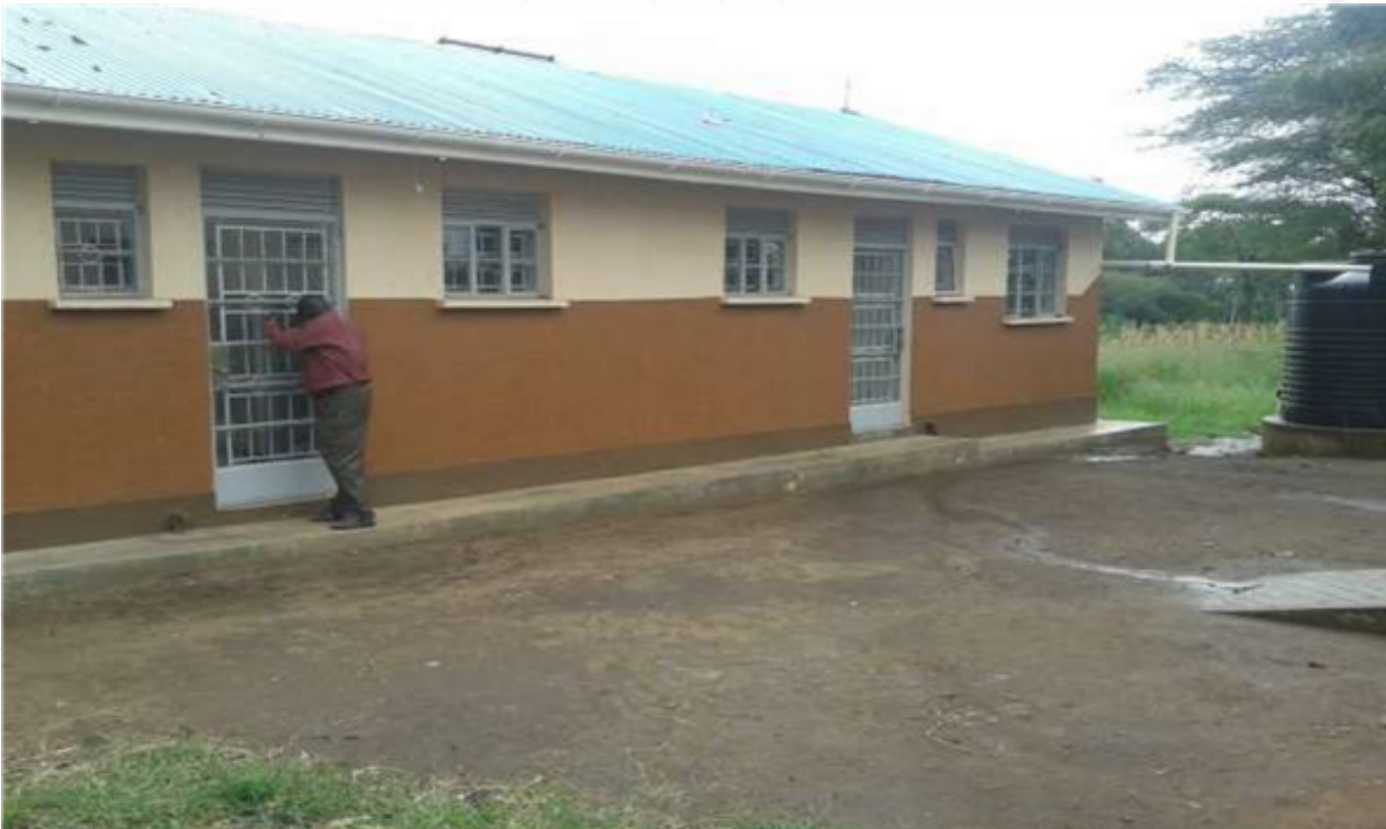
Fig 5: Completed staff house at tapac Health Centre III- Moroto District under NUSAF project – Office of the Prime Minister.
